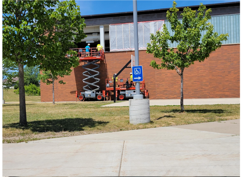
MS Pool window replacement
